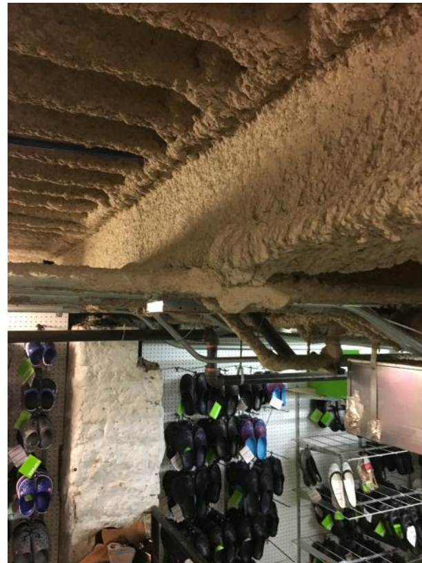
5 CELLAR DATE TAKEN 06/14/2017 TAKEN FROM SOUTH SIDE LOOKING NORTH
