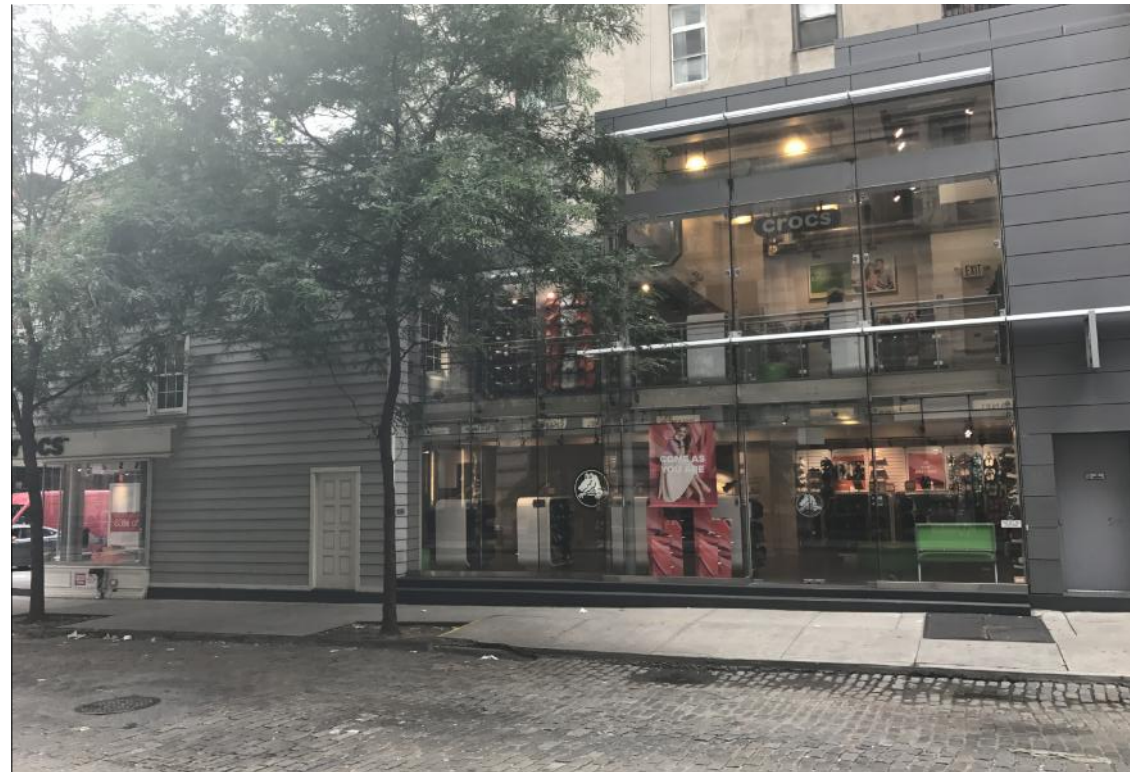
1 143 SPRING STREET DATE TAKEN 07/06/2017 TAKEN FROM EAST SIDE OF WOOSTER LOOKING SOUTHWEST
