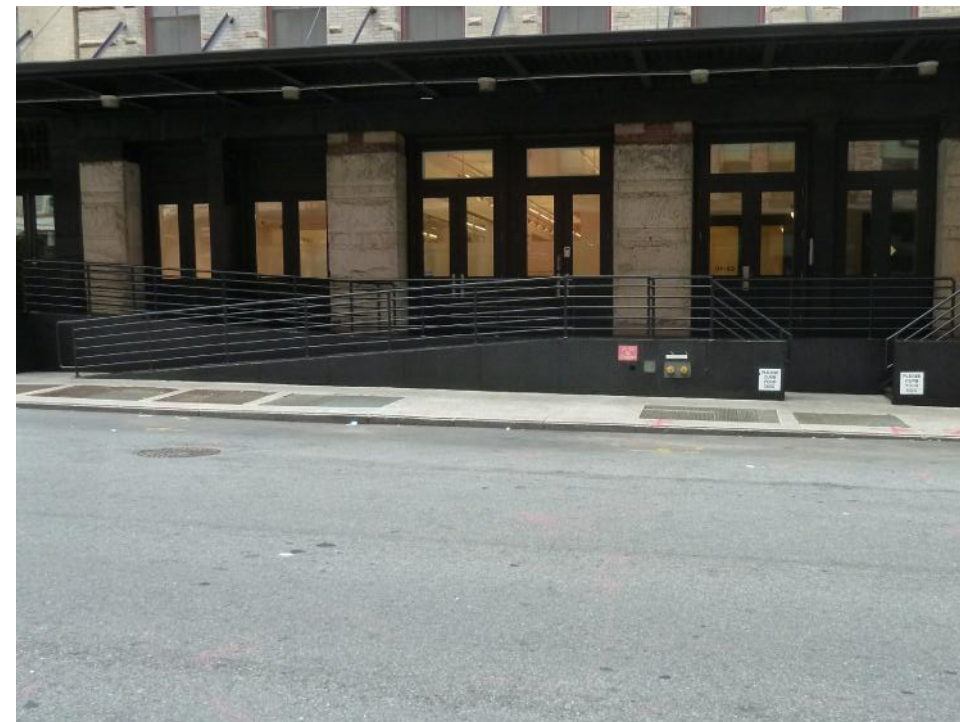
31 NORTH MOORE STREET TRIBECA WEST HISTORIC DISTRICT
