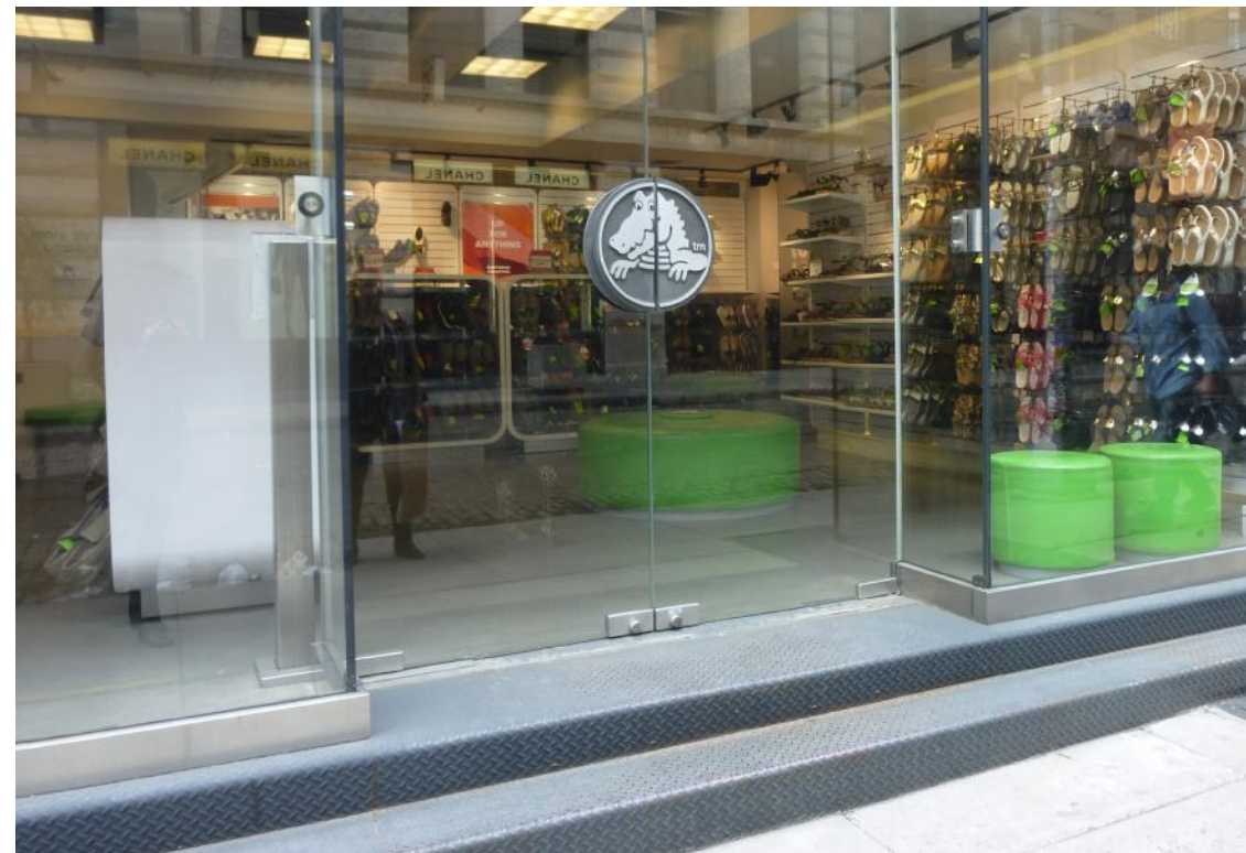
4 143 SPRING STREET DATE TAKEN 04/14/2017 CLOSE UP OF WOOSTER STREET ENTRY STAIR
