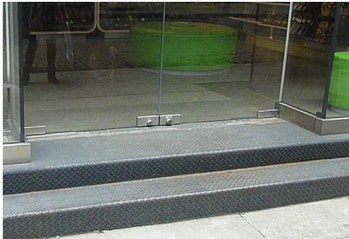
3 143 SPRING STREET DATE TAKEN 04/14/2017 CLOSE UP OF WOOSTER STREET ENTRY STAIR
