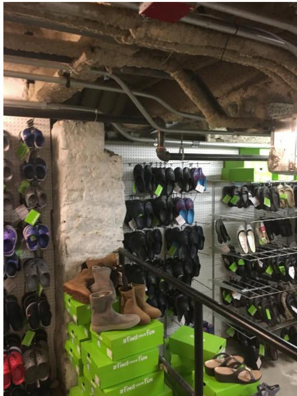
4 CELLAR DATE TAKEN 06/14/2017 TAKEN FROM SOUTH SIDE LOOKING NORTH
